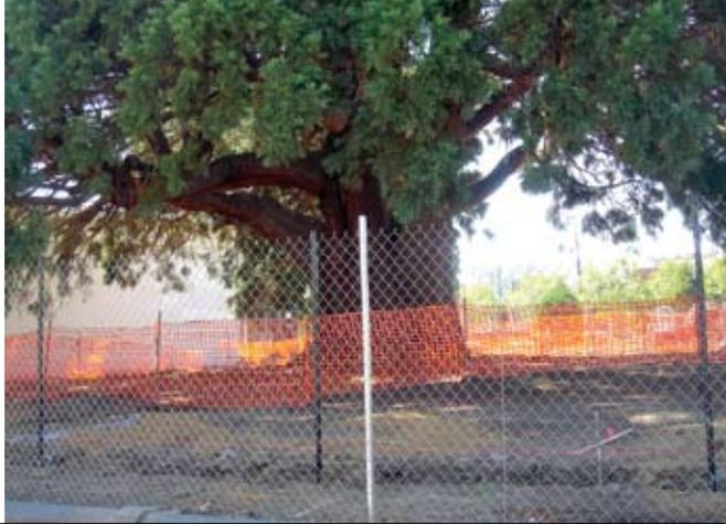
**Ideal Fencing Materials:** Trees to be preserved may be protected with five or to six (5' - 6') foot high fences. Fences are to be mounted on two-inch diameter galvanized iron posts, driven into the ground to a depth of at least 2-feet at no more than 10-foot spacing. Paved areas: if fencing must be located on paving or concrete that will not be demolished, the posts may be supported by an appropriate grade level concrete base.
